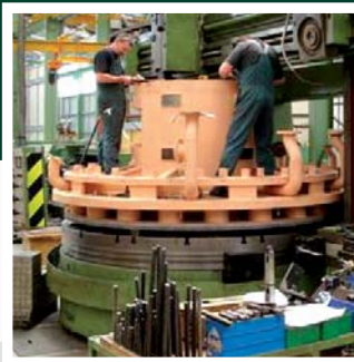
Repair, refurbishment and assembly of Head Covers
