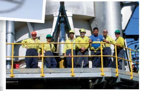
Design, manufacture and installation of Washer Diffuser Upgrade to increase stroke and capacity
